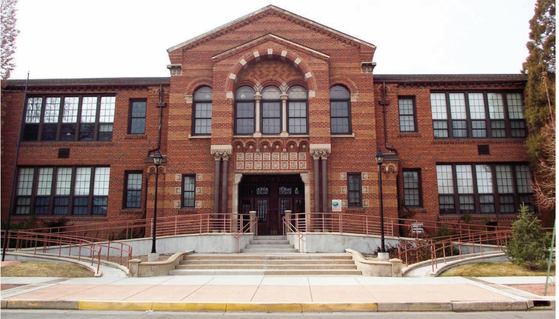
**Figure 9.2.** The school district instructed architect Walter DeMordaunt to modify his Carlile School building design for the Bessemer School, above, using brick instead of stucco and with slight modification on structural design. (*Jeffrey DeHerrera*)
