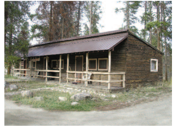
Figure 3.5. Building 5 (Units 10-12, “The Bunk House”) Thomas
