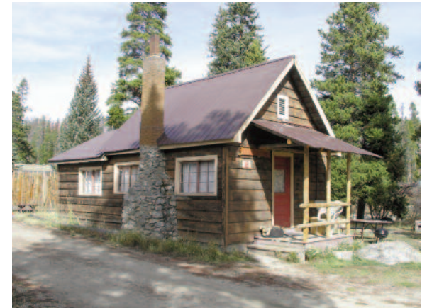
Figure 3.1. Building 1 (Unit 6, “Mossridge” Cottage) Thomas
