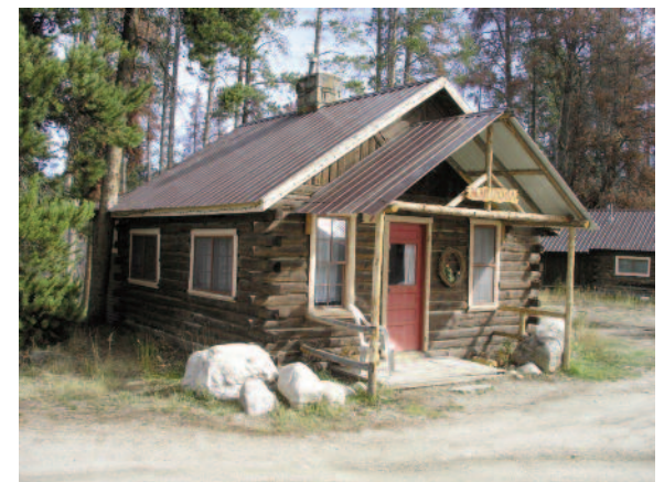
Figure 3.2. Building 2 (Unit 7, “Mariposa” Cottage) Thomas
